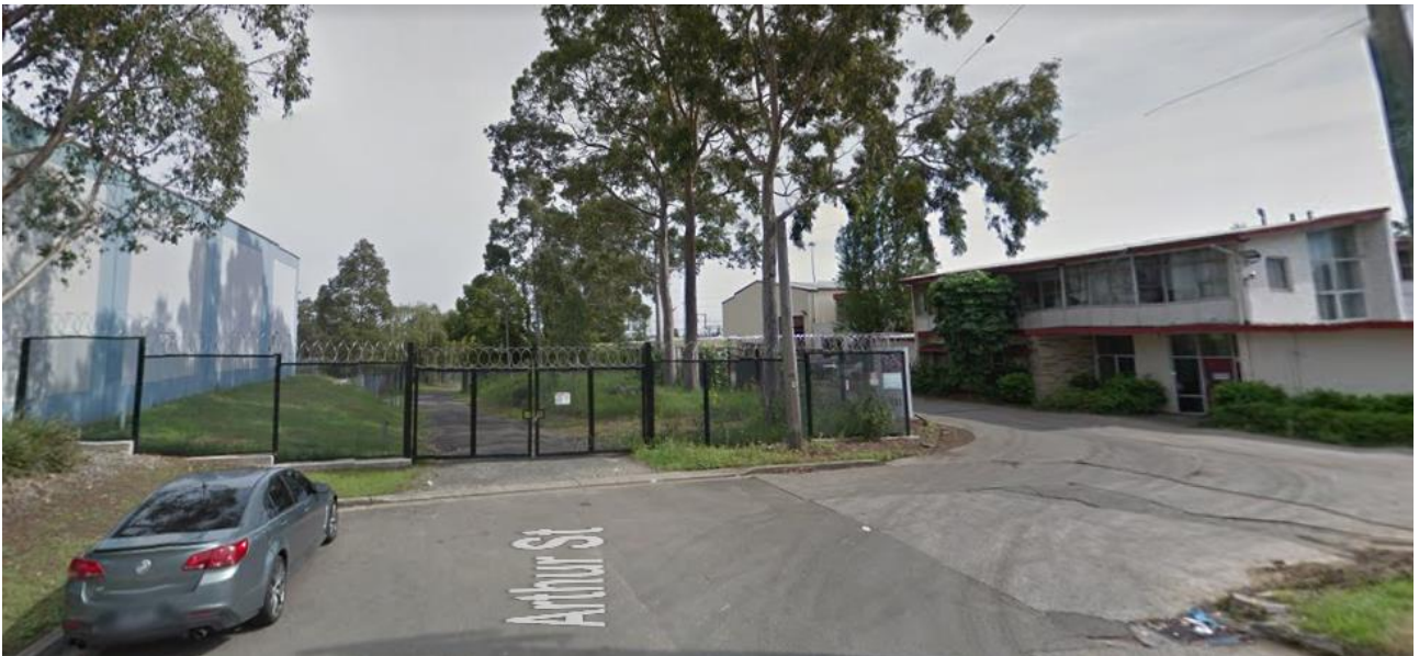
Figure 5. Main entry to the subject site at the western end of Arthur Street. The existing 9m wide driveway crossing is to be retained.
